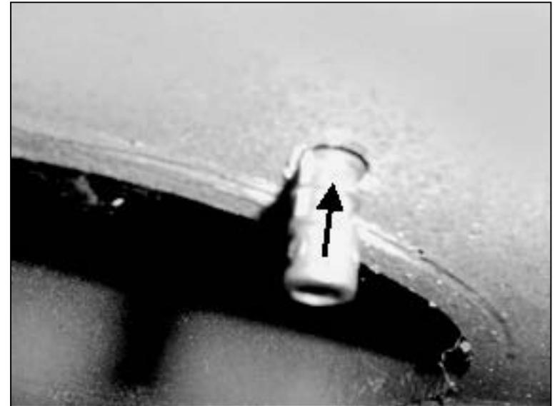
Insert the lag shields flush to the wall.
