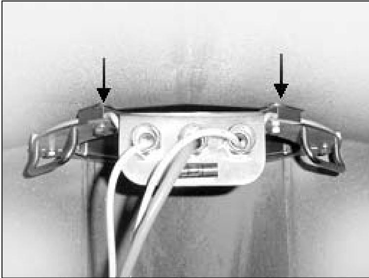
If installing the Cartridge in a round manhole, it may be necessary to use flat washers as spacers between the Cartridge flange and the wall.
