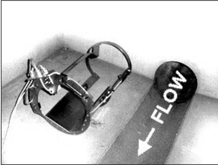
The Cartridge should be installed in the incoming pipe of the manhole.
