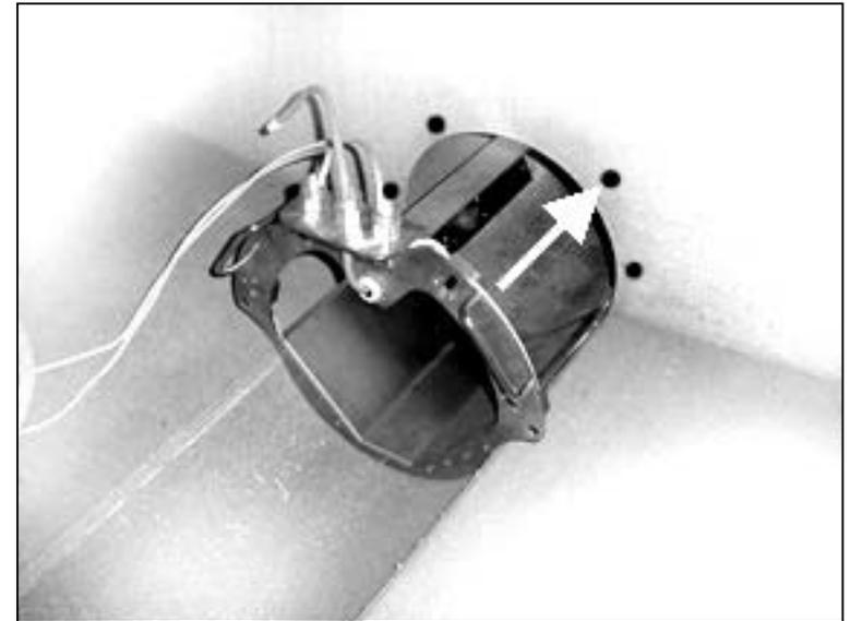
Re-insert the Cartridge. Line up the slots with the lag shield holes and screw the lag bolts with the flat washers through the flange in the Cartridge and snug tight.
