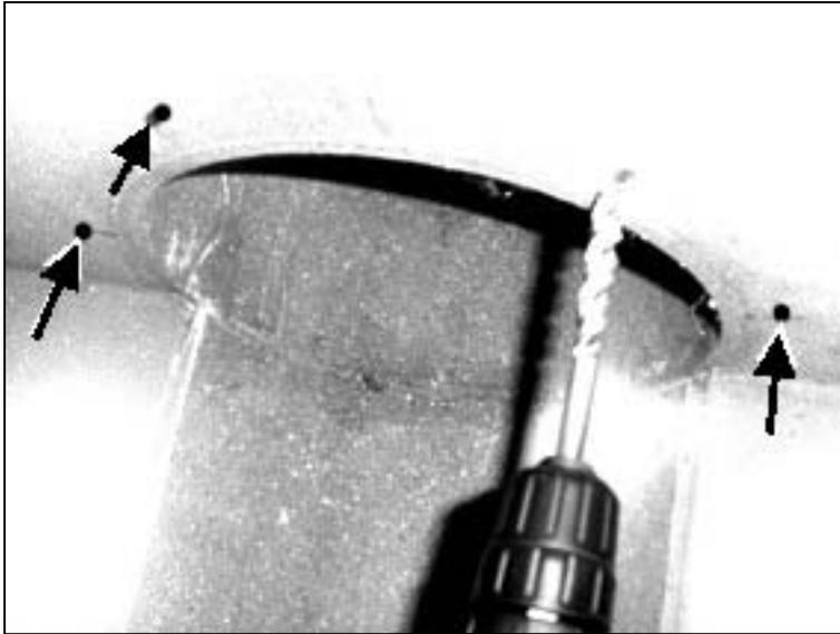
Using the drill and the masonry drill bit provided, drill all four holes for the lag shield.
