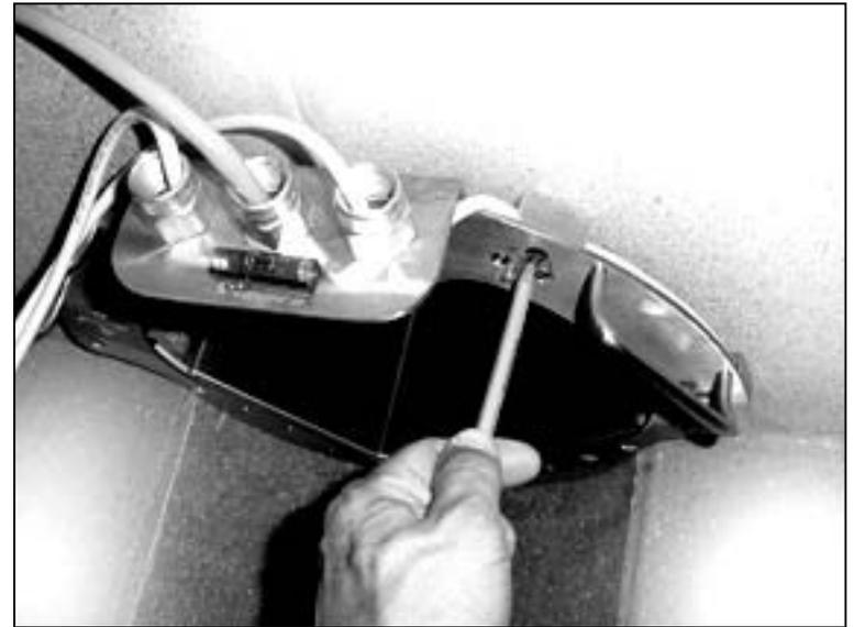
Use a pencil or marker and mark the four slotted holes provided in the flange of the Cartridge. Remove the cartridge from the pipe.
