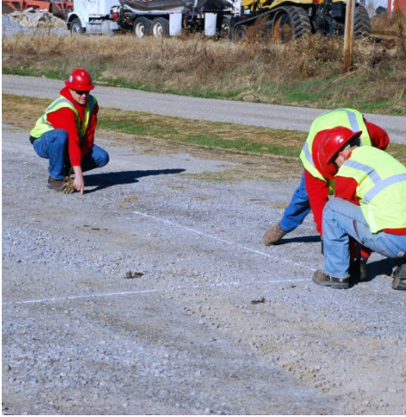
Step 1: Choose site with flat and level approaches twice the length of your longest truck
