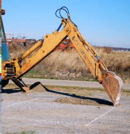
Step 2: Excavate and compact 14 X 10 foot hole 2 feet deep. Dig trench for home run cable and drains
