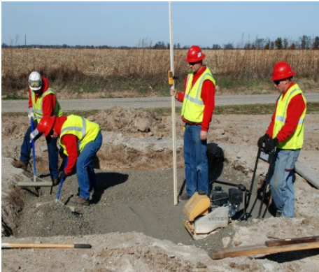
Step 4: Lay second layer of stone, compact flat and level. Surface should be 11.5 inches below grade
