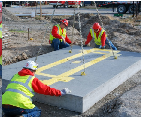
Step 6: Set the scale using 50' of masons twine to ensure it is parallel to the road
