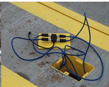
Step 8: Make watertight electrical connections at scale and controller. Back fill perimeter of scale, drains and conduit runs
