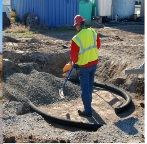
Step 3: Lay 4" tile drain and first 6 inch layer of CA6 crusher run stone. Compact to 95%
